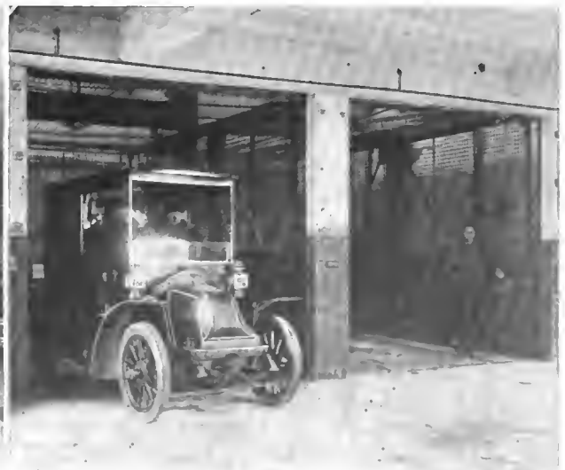
LIFTS THAT CARRY THE LARGEST CARS.
